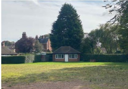
Old tennis pavilion with toilets
